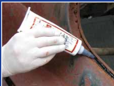
Squeeze a bead of POR PATCH™ into seam.
